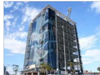
exterior Cristec Vipla SI Project > Murcia, Spain
